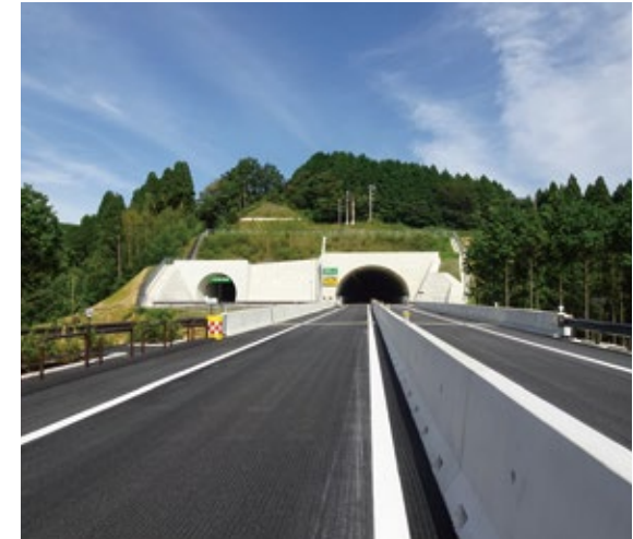
Futae-no-toge Mountain Pass Tunnel (Kumamoto Prefecture)
