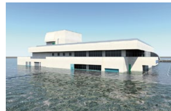
Examination of water resistance (inundation simulation) at Asahikawa City Sewage Treatment Center (Hokkaido)
