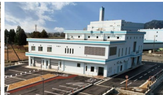
Chuo Waste Treatment Centre (Akita Prefecture)
