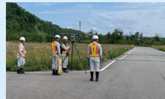
Surveying for disaster restoration of town roads (Ishikawa Prefecture)
