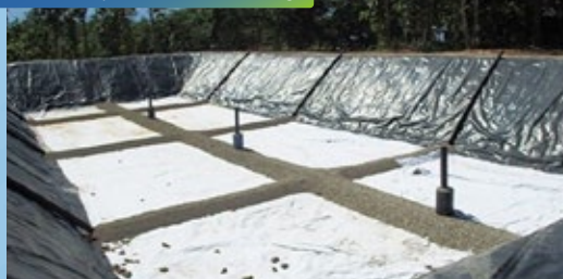
Semi-aerobic landfill project harnessing microbial power to reduce methane emissions and lessen environmental impact (Thailand)
