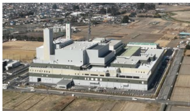
Minuma Environmental Centre - waste incineration and recycling facility (Saitama Prefecture)
