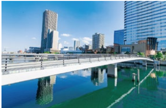
Sakurakobashi Footbridge (Tokyo)
