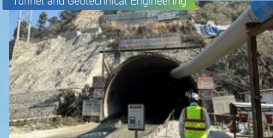
Design, construction, and supervision of Nagdhunga Tunnel (Nepal)
