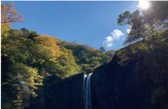
Daijizawa No. 1 Sabo Dam (Tochigi Prefecture)
