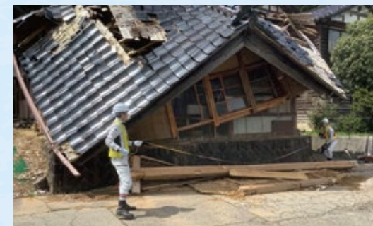
Publicly funded demolition survey (Ishikawa Prefecture)
