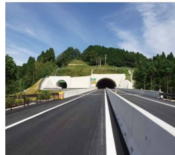
Futae-no-toge Mountain Pass Tunnel (Kumamoto Prefecture)
