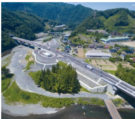
PPP initiative to accelerate the Sanriku Coastal Road Project (Iwate Prefecture)
