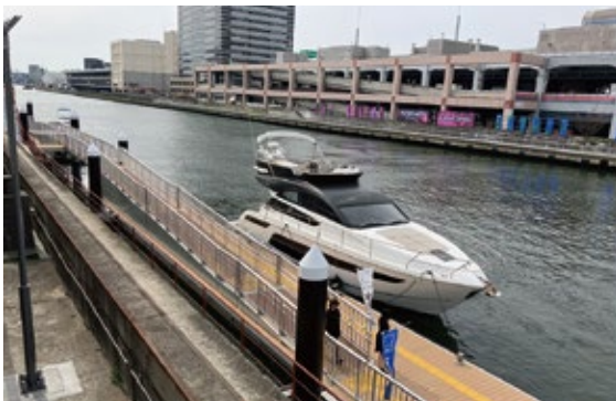
Nakanoshima GATE South Pier (Osaka Prefecture)
