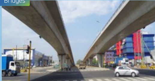
Nyerere Road flyover project linking Dar es Salaam city centre with the international airport (Tanzania)
