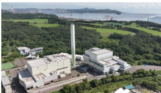
Nishi Iburi Eco Factory - refuse incineration facility (Hokkaido)
