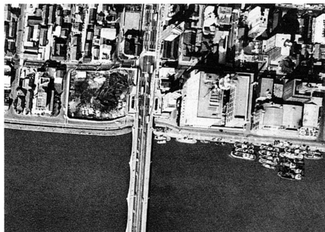
Photo 3-3 Revetment near Bandai Bridge on the Shinano River
