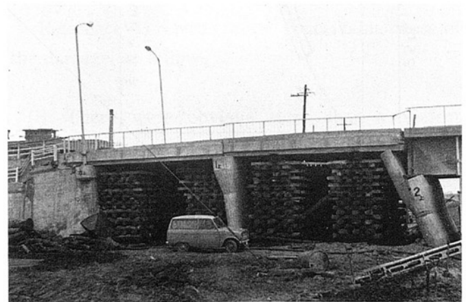
Photo 3-7 Damage to the abutment and the piers of Yachiyo Bridge on the left bank
