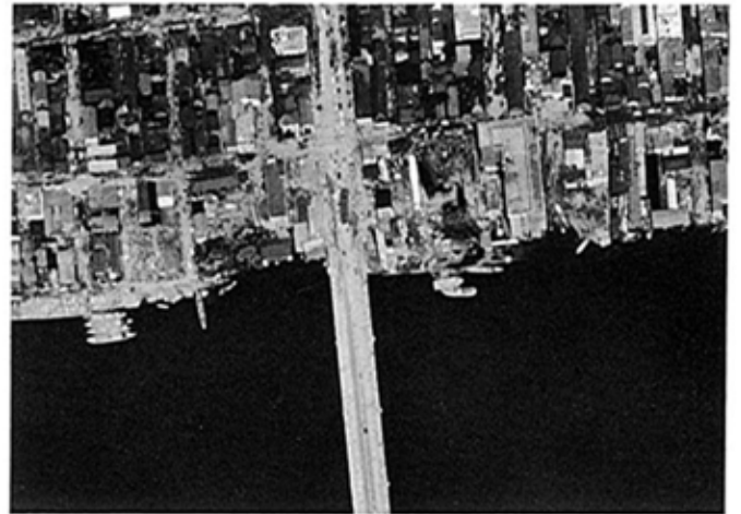
(b) After the earthquake
