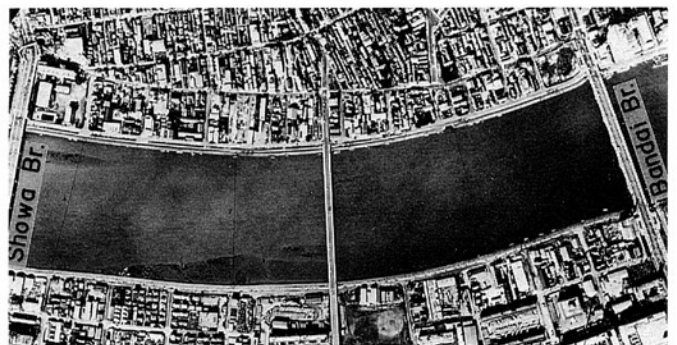
(b) After the earthquake (1971)
