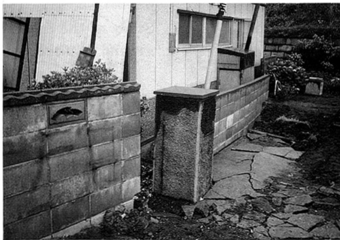
Photo 2-7 Cracks with subsidence on the northern slope of Mae Hill (Courtesy of Prof. Y. Mori, Nihon Univ.)
