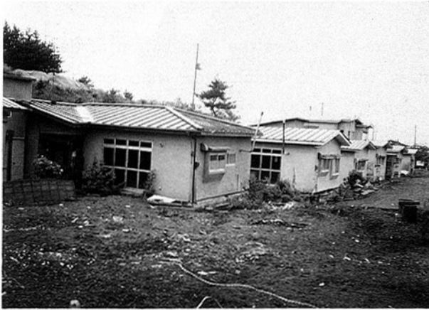
Photo 2-6 Undulating ground on the northern slope of Mae Hill (Courtesy of Prof. Y. Mori, Nihon Univ.)
